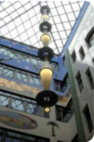
Shopping Arcade Renovation, Leipzig, Germany
